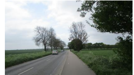
View of the existing route
