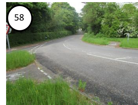
View towards Swaffham Prior with slip road (57) emerging on left. Note jug handle arrangement on right of picture and space available in carriageway for refuge.
