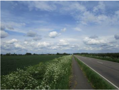
The existing narrow path.
