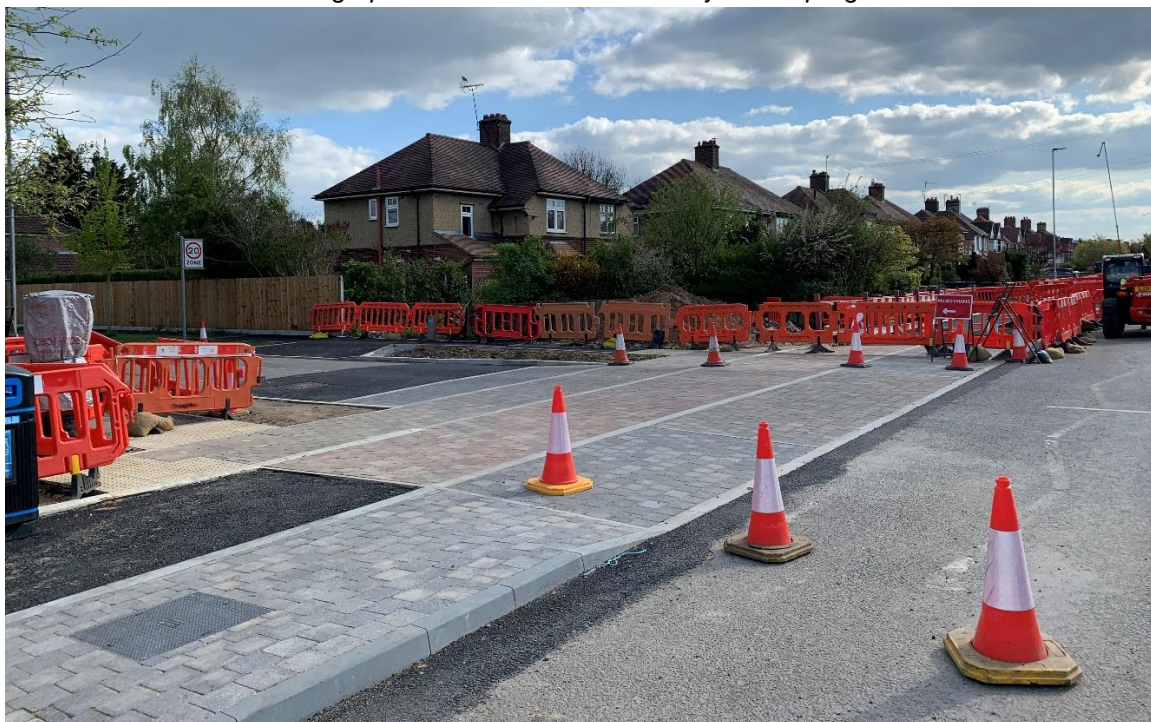
*Photograph shows Kendal Way junction progress
