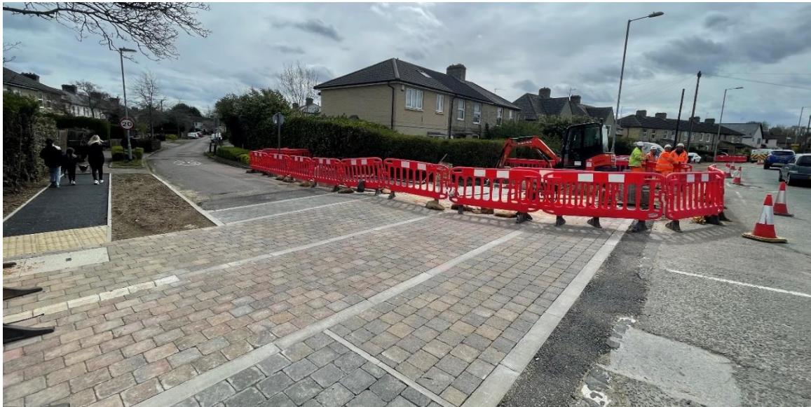
*Photograph shows Oak Tree Avenue junction progress
