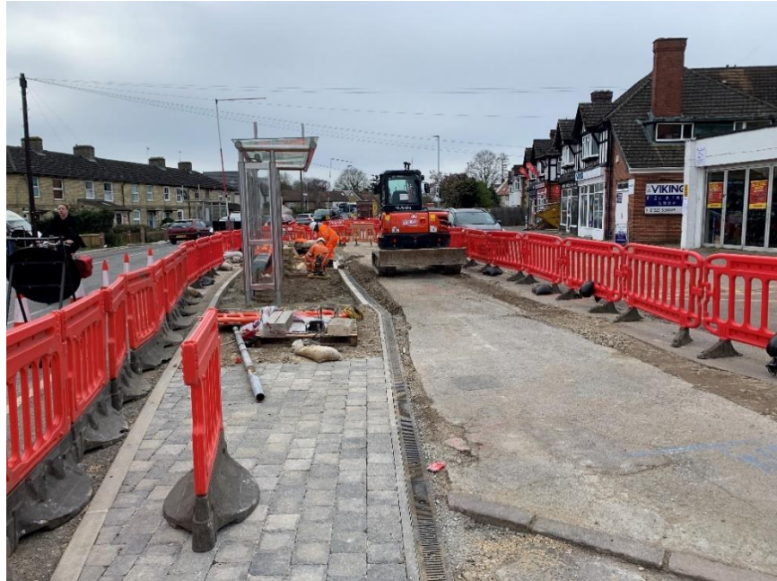
Block paving being laid at the Arbury Road shops
