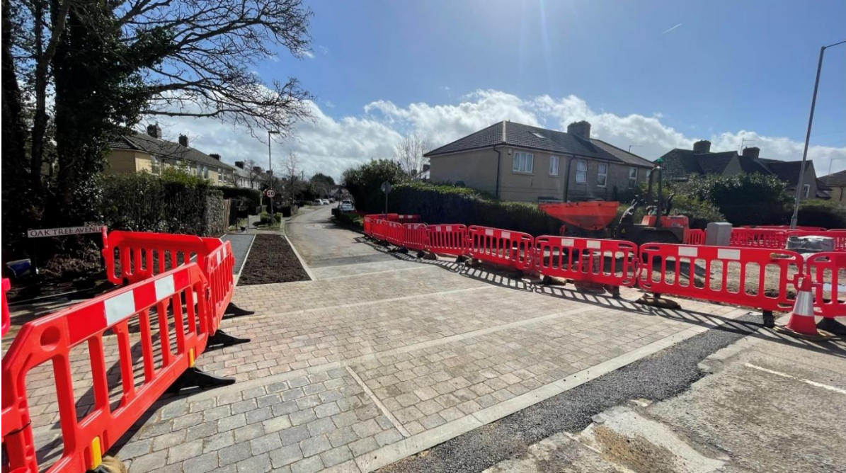
*Photograph shows Oak Tree Avenue junction progress
